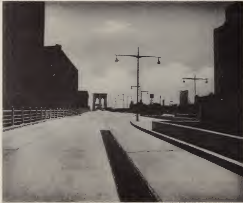
The completed north roadway was opened to traffic on Sept. 30, 1953. This is the beginning of the Manhattan Plaza.
